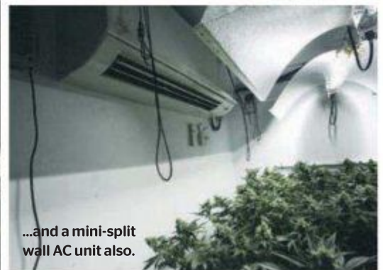
A filter and fan fit in this closet garden...
